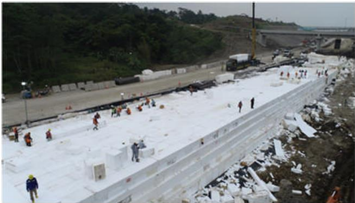
EPS Geofoam in use for slope stabilization in West Java, Indonesia.
