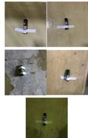
Figure 3.13. The installation of accelerometers for the purpose of recording vibration data.
